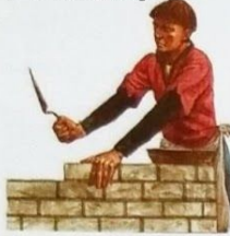
Roughmasons placed the stones in the wall, according to the numbers put on them by the masons.
