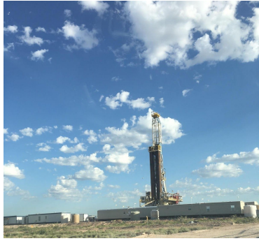
Rig behind the housing for the crew and companymen
