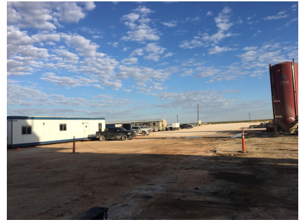
Another shot of the crew's trailers.
