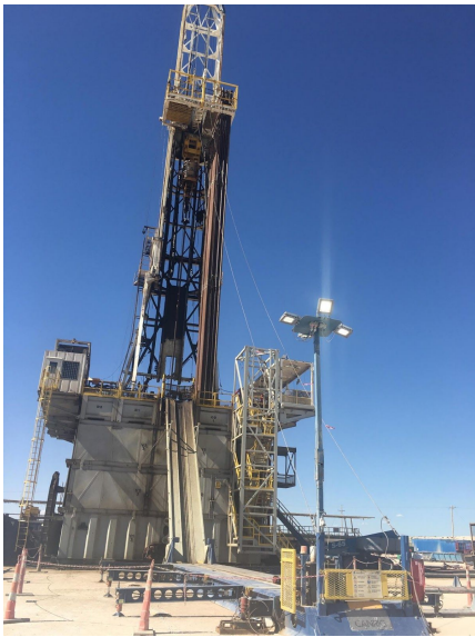
Front of the rig. The blue machine is what brings up the drill pipe. It is called a pragma
