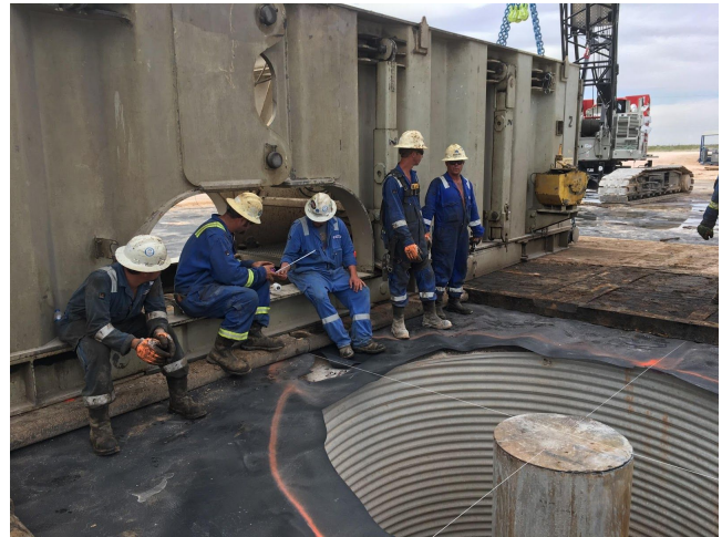
The drilling hole, before the rig goes on it.
