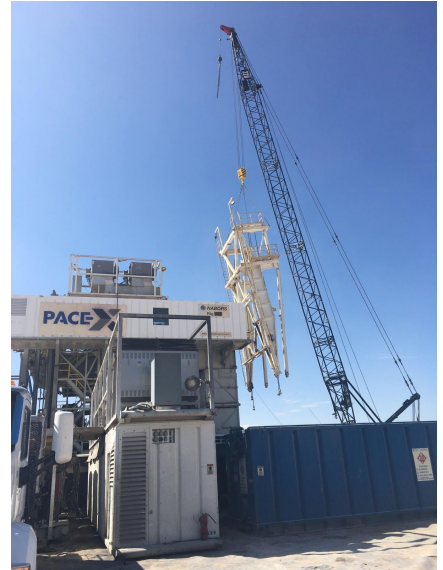
A crane taking rig apart after drilling is done.
